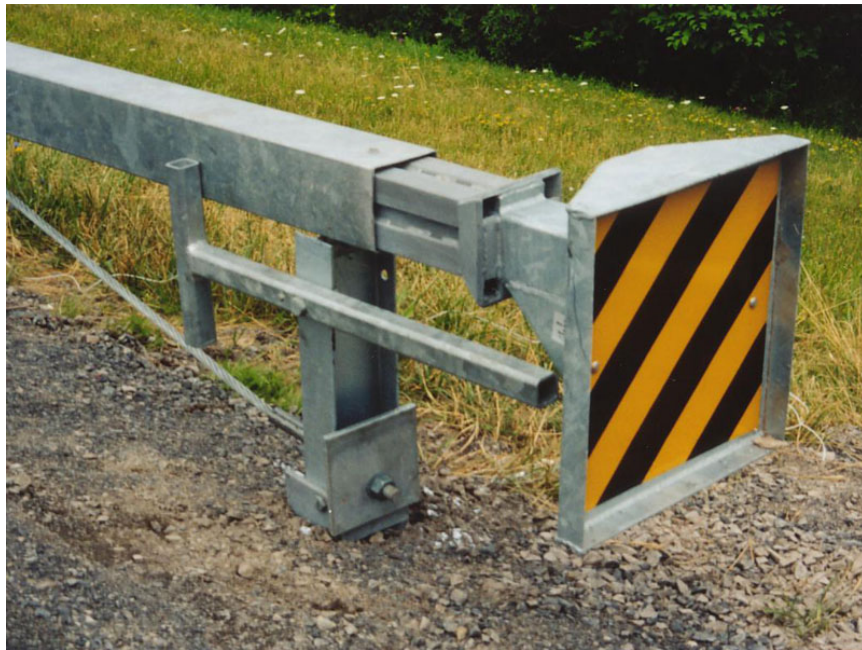
A W-BEAM to BOXBEAM guardrail connection
