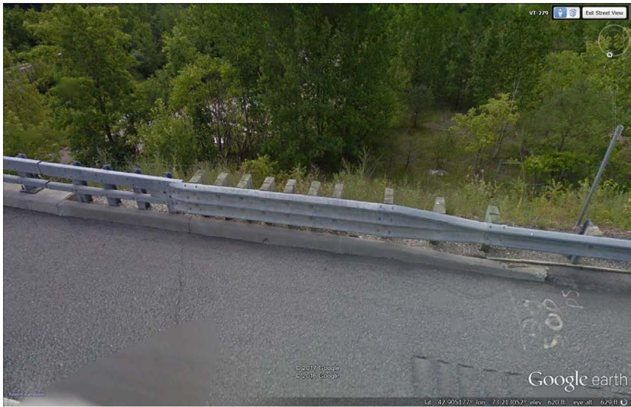
A Thriebeam bridge approach terminal installed with wood posts
